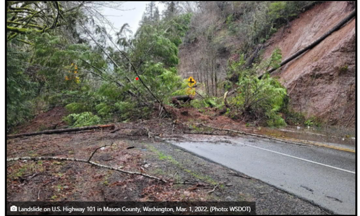
Landslide on U.S. Highway 101 in Mason County, Washington, Mar. 1, 2022. (Photo: WSDOT)
