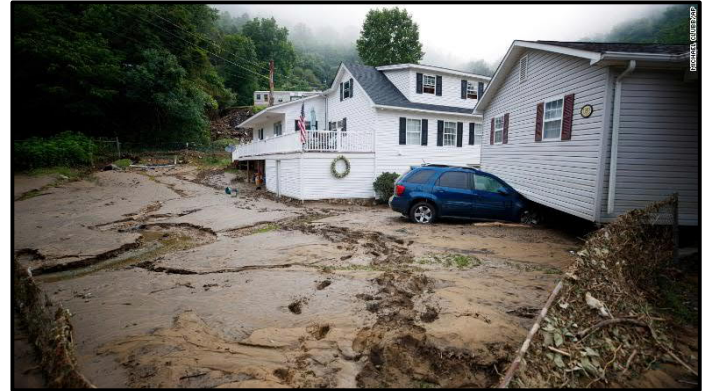
A house was moved off its foundation after a flash flood, Thursday, July 14, 2022, in Whitewood, Virginia.
